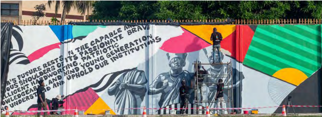
A work-in-progress photo of the graffiti mural at the famous Ozumba Mbadiwe Street in Lagos. The 3 statues of Lagos state are ably displayed creatively.
