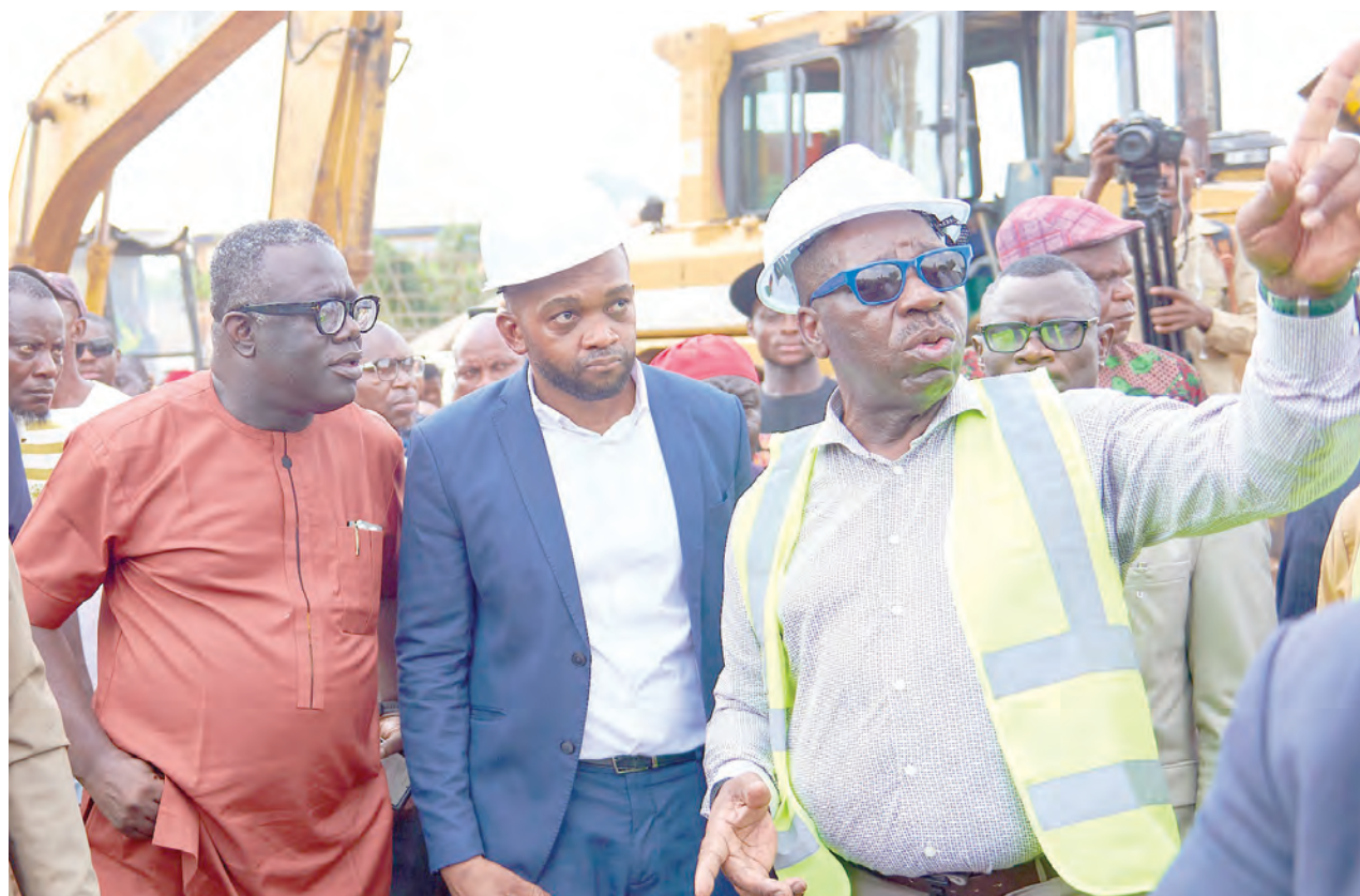
L-R: Tom Obaseki, executive chairman, Oredo Local Government Area (LGA), Edo State; Ethan Uzamer, commissioner for roads and bridges; and Godwin Obaseki, governor, during the flag-off of the construction of 20km Iyekogba Road, in Oredo LGA, in Edo State, recently.
