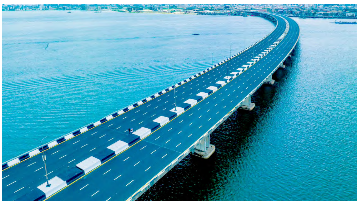
The reopening of the Third Mainland Bridge after a three-month partial closure for extended repair works.
